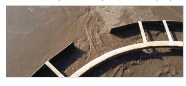
Designed for torque requirements from 1,000 ft-lbs to 6,000,000 ft-lbs, the Premium Drive Unit provides rotational force to the clarifier mechanism while resisting torque loads and overturning moments.
